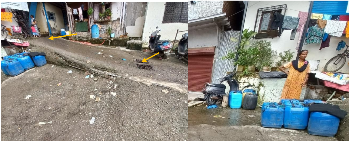
All the water from the huts area flows through the ground
