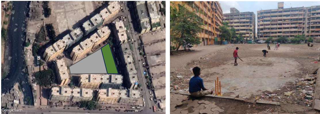
Figure 3.10 Concretization of the maidan. Grey colour indicated zone in above image shows the concretised portion of maidan. Image highlighting the concretised areas of maidan. This is a 6" slab of previously existing structure which is kept as it is and not demolished, leading to a lack of water absorptive surface area in this part.
